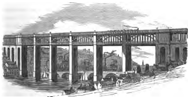
THE HIGH-LEVEL BRIDGE AT NEWCASTLE.
